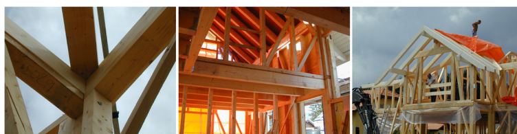
Figure 1 Structures built by carpenters. Examples of such structures.
